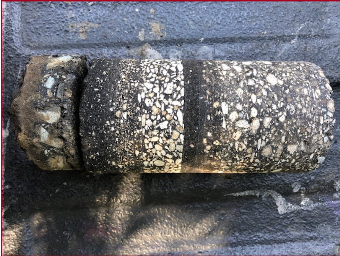
FIGURE 5A: PHOTOGRAPH OF PAVEMENT CORE AT P-1
